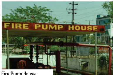
Fire Pump House
