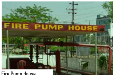
Fire Pump House
