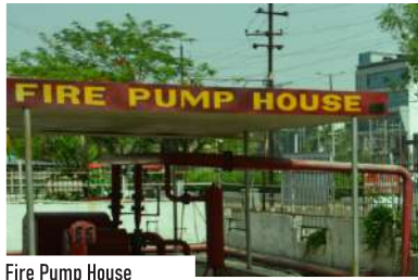
Fire Pump House
