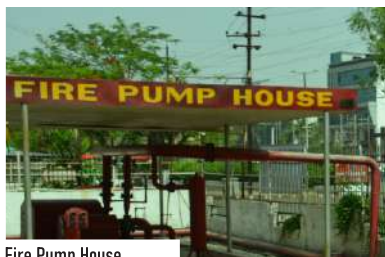
Fire Pump House
